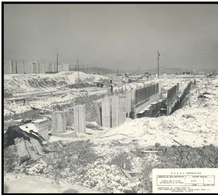
Figure 6: Looking North at the X-705 Decontamination Building Site, December 1953
