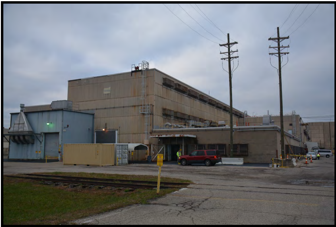
Figure 4: South Side of the X-705 Decontamination Building, November 2014, Facing Northwest
