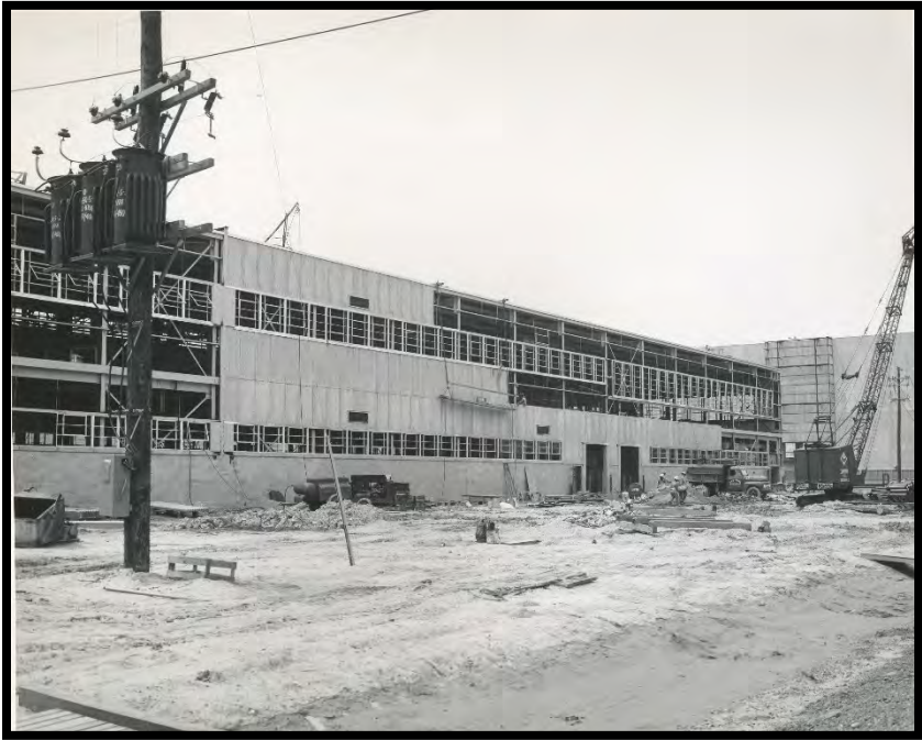
Figure 18: The X-705 Decontamination Building, July 1954
