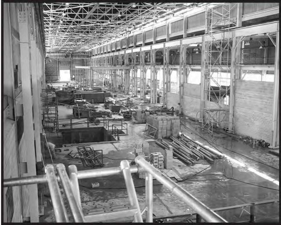
Figure 19: Interior View of the X-705 Decontamination Building, July 1954
