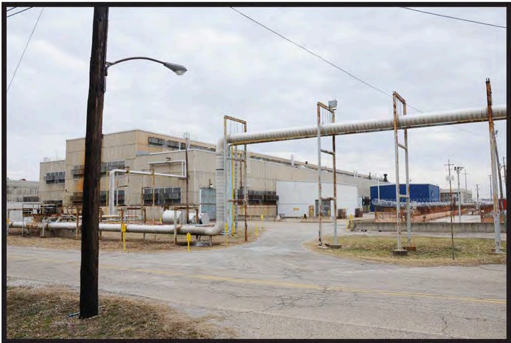
Figure 2: North Side of the X-705 Decontamination Building, August 2014, Facing Southeast
