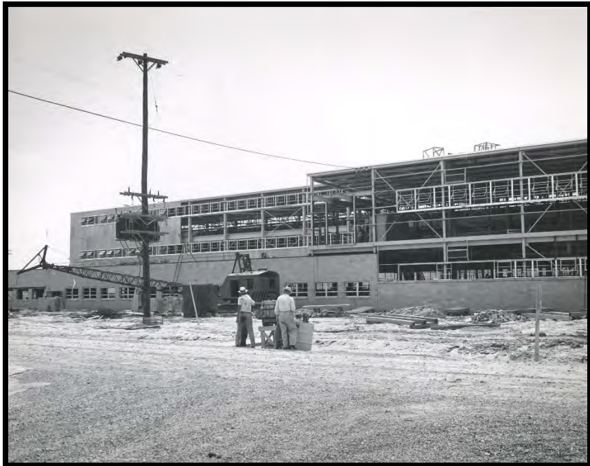
Figure 14: The X-705 Decontamination Building, July 1954
