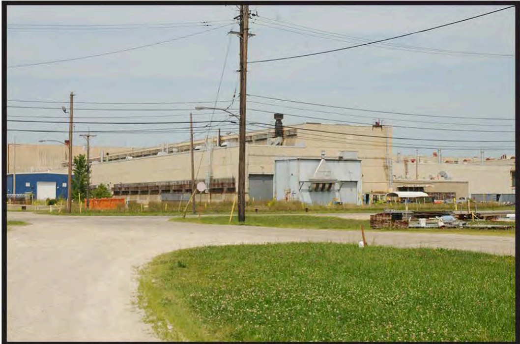
Figure 3: South Side of the X-705 Decontamination Building, August 2014, Facing Northeast
