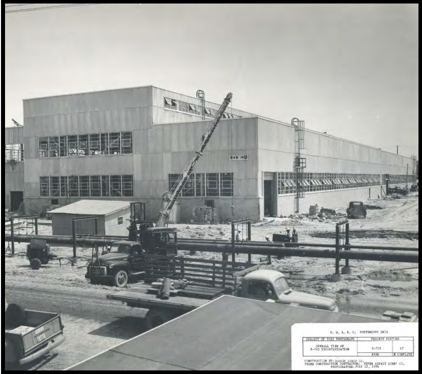
Figure 17: Overall View of the X-705 Decontamination Building, Looking North, July 1954
