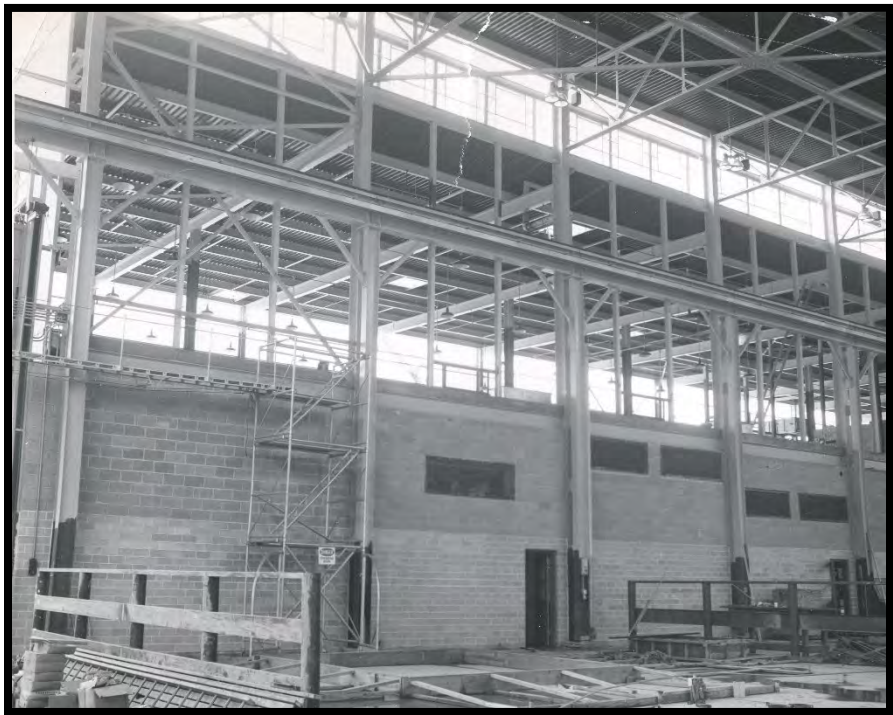
Figure 15: Interior View of the X-705 Decontamination Building, July 1954
