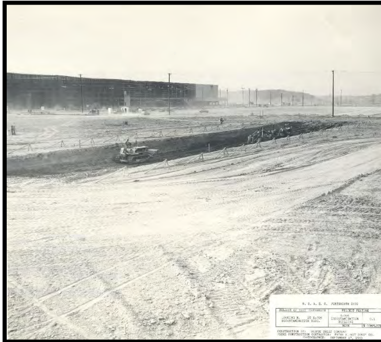
Figure 5: Interior View of the X-705 Decontamination Building Site, Looking North, September 1953
