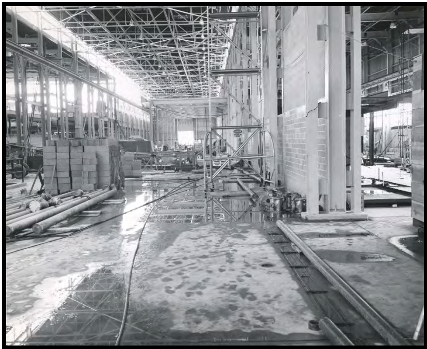
Figure 13: Interior View of the X-705 Decontamination Building, July 1954
