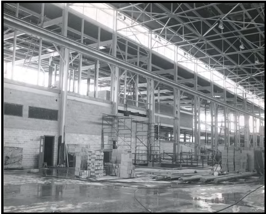
Figure 16: Interior View of the X-705 Decontamination Building, July 1954
