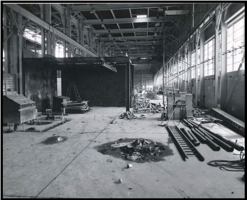
Figure 12: Interior View of the X-705 Decontamination Building, July 1954
