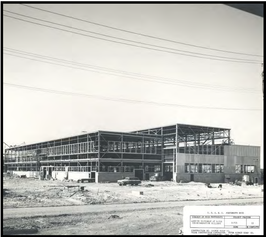
Figure 11: Looking Southwest at the X-705 Decontamination Building, June 1954
